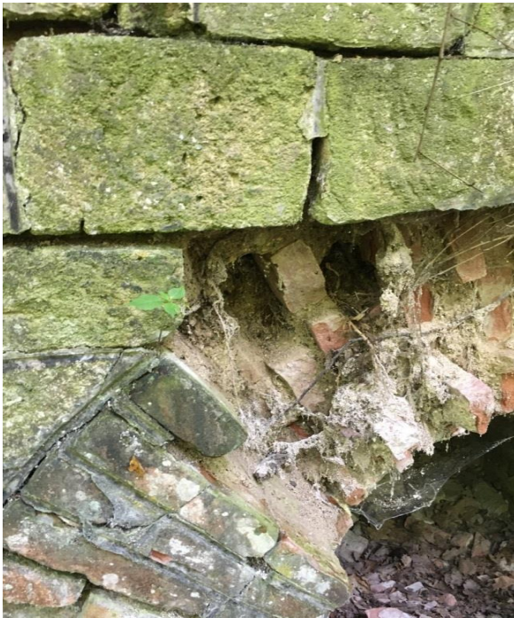
Obr.283 Detail klenby propusti
