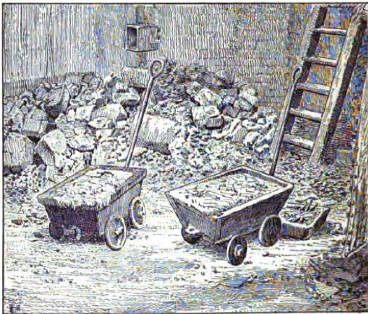
Fig. 68.—Tapping cinder from ball furnace.
