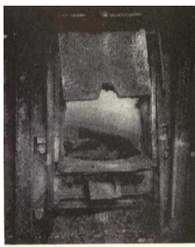
Fig. 7.—Pig Iron in Puddling Furnace.
